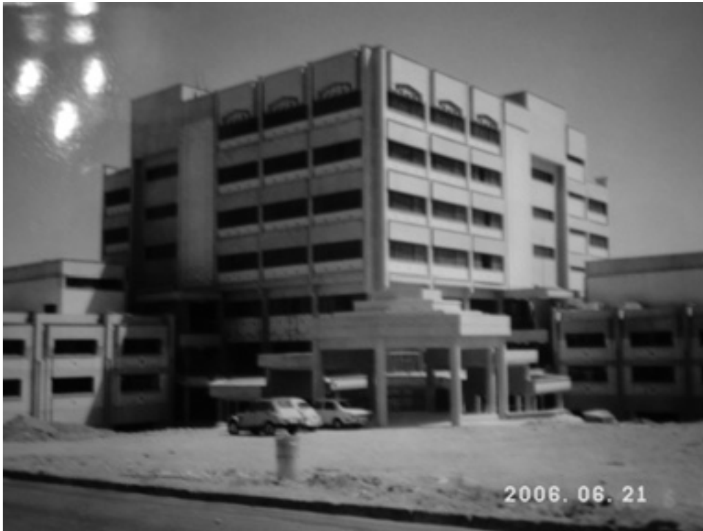
Isfahan University Library Building
